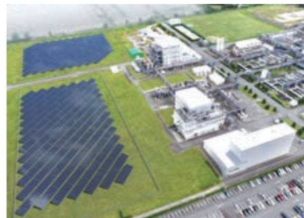
Daiichi Sankyo Chemical Pharma Onahama Plant: concept drawing of the onsite solar power system following completion
