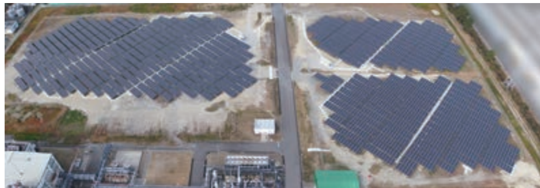
Onahama Plant: the onsite solar power system
