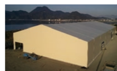
Depressurized tent to prevent scattering
