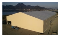
Depressurized tent to prevent scattering
