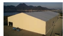
Depressurized tent to prevent scattering
