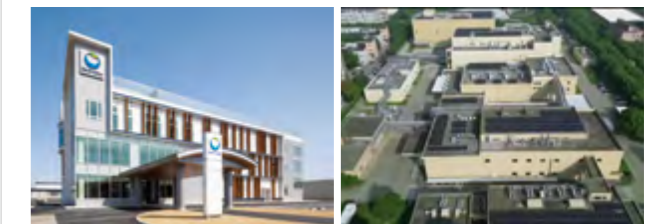
Onahama Plant Administration Building | Solar panels seen from the roof of the Shanghai plant
