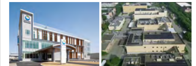
Onahama Plant Administration Building | Solar panels seen from the roof of the Shanghai plant
